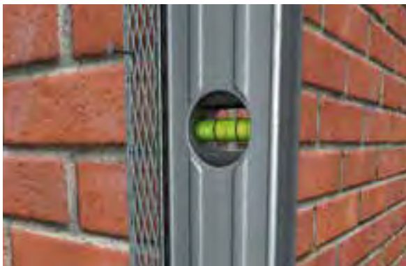
■ ENSURING THE BEAD IS PLUMB AND STRAIGHT
