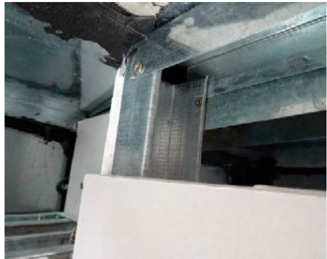
■ STEEL STUD FIXED INTO HEAD TRACK
